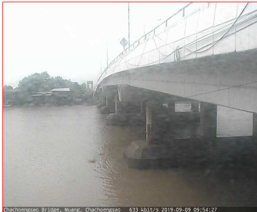
Chachoengsao Bridge, Muang, Chachoengsao 633 kbit/s 2019-09-09 09:54:27
