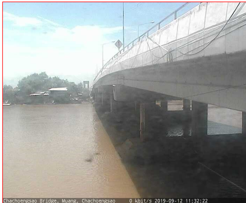
Chachoengsao Bridge, Muang, Chachoengsao 0 kbit/s 2019-09-12 11:32:22
