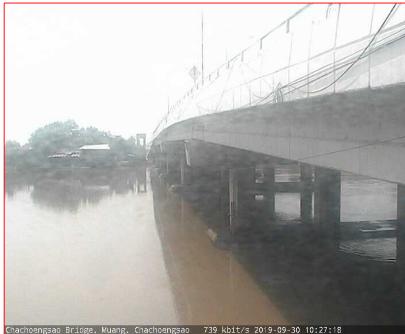
Chachoengsao Bridge, Muang, Chachoengsao 739 kbit/s 2019-09-30 10:27:18
