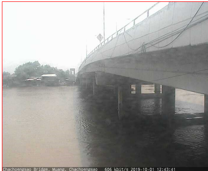
Chachoengsao Bridge, Muang, Chachoengsao 606 kbit/s 2019-10-01 12:43:41
