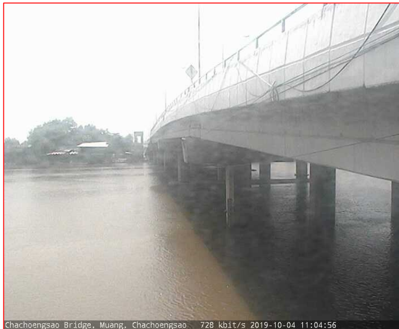
Chachoengsao Bridge, Muang, Chachoengsao. 728 kbit/s 2019-10-04 11:04:56
