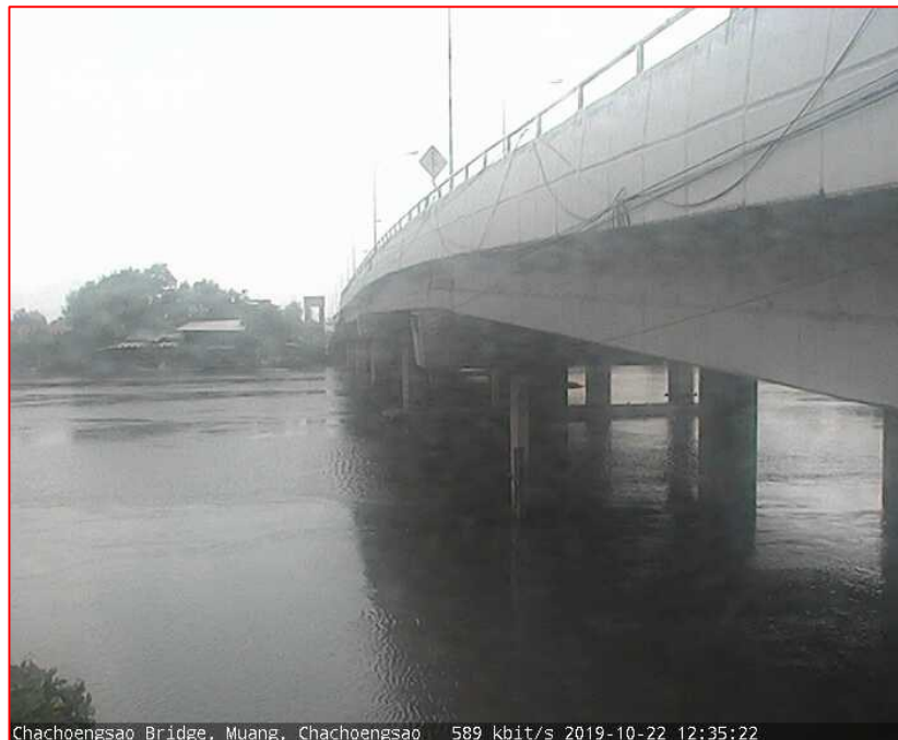
Chachoengsao Bridge, Muang, Chachoengsao 589 kbit/s 2019-10-22 12:35:22
