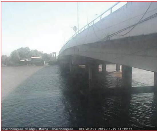
Chachoengsao Bridge, Muang, Chachoengsao 701 kbit/s 2019-11-25 14:39:37
