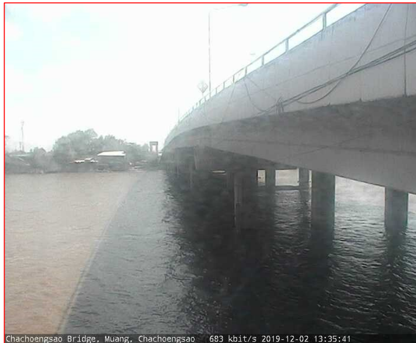
Chachoengsao Bridge, Muang, Chachoengsao 683 kbit/s 2019-12-02 13:35:41
