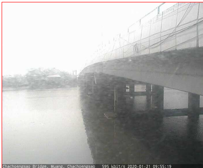
Chachoengsao Bridge, Muang, Chachoengsao 595 kbit/s 2020-01-21 09:55:19
