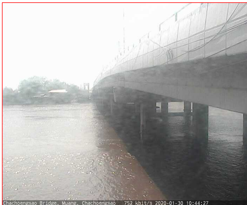
Chachoengsao Bridge. Muang, Chachoengsao 752 kbit/s 2020-01-30 10:44:27
