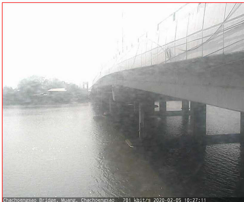
Chachoengsao Bridge. Muang, Chachoengsao 701 kbit/s 2020-02-05 10:27:11
