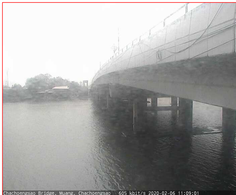
Chachoengsao Bridge. Muang, Chachoengsao 605 kbit/s 2020-02-06 11:09:01
