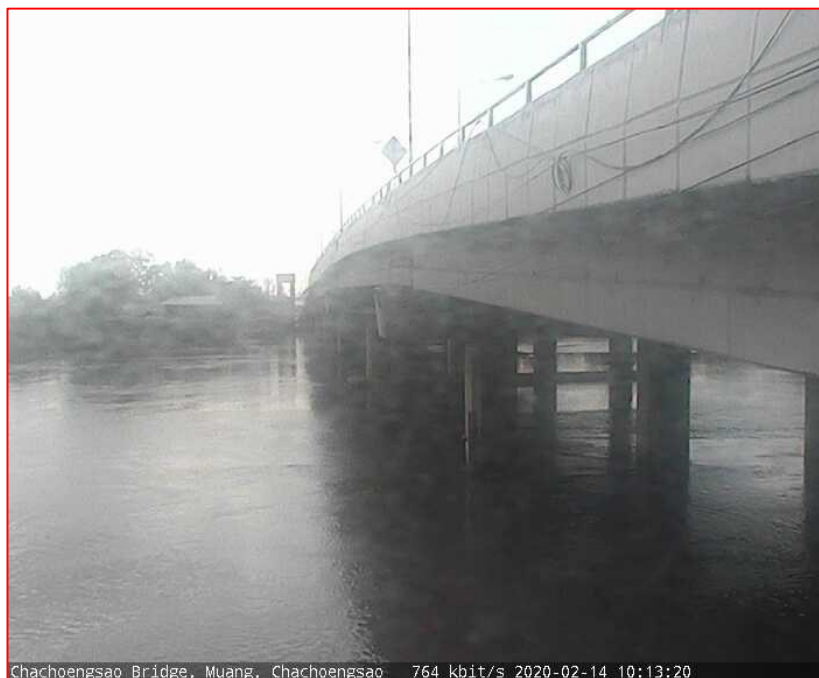
Chachoengsao Bridge, Muang, Chachoengsao 764 kbit/s 2020-02-14 10:13:20
