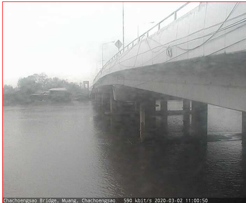
Chachoengsao Bridge, Muang, Chachoengsao 590 kbit/s 2020-03-02 11:00:50
