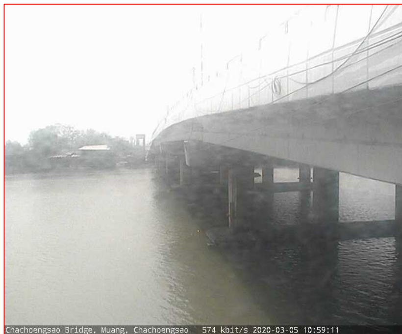
Chachoengsao Bridge. Muang, Chachoengsao 574 kbit/s 2020-03-05 10:59:11
