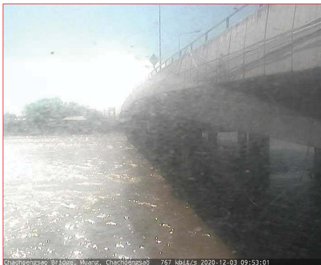
Chachengsao Bridge, Muang, Chachengsao 767 kb.t/s 2020-12-03 09:53:01
