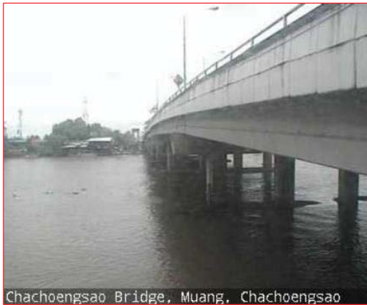
Chachoengsao Bridge, Muang, Chachoengsao
