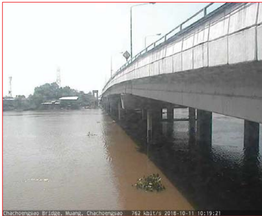
Chachoengsao Bridge, Muang, Chachoengsao 762 kbit/s 2018-10-11 10:19:21
