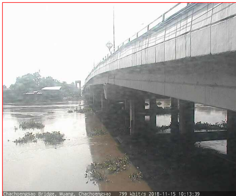
Chachoengsao Bridge, Muang, Chachoengsao 799 kbit/s 2018-11-15 10:13:39
