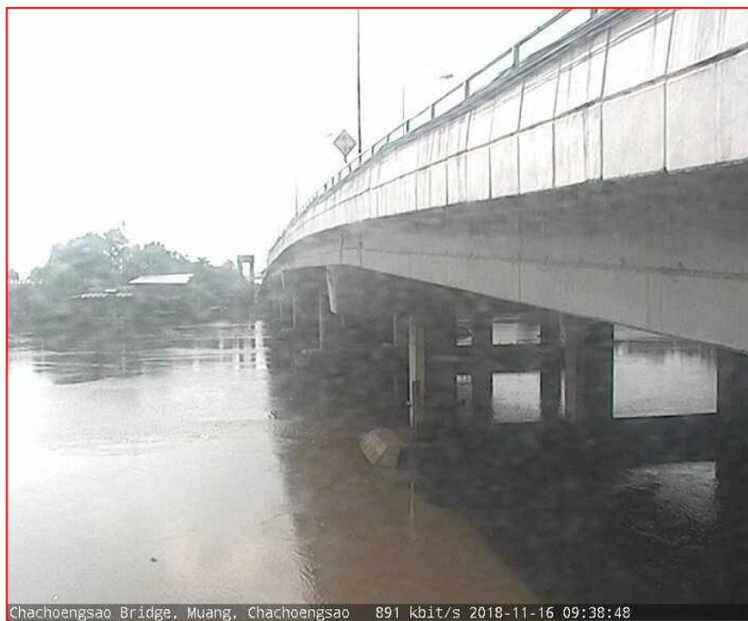
Chachoengsao Bridge, Muang, Chachoengsao 891 kbit/s 2018-11-16 09:38:48
