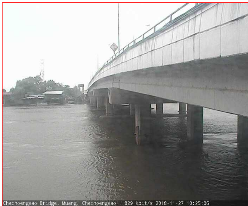
Chachoengsao Bridge, Muang, Chachoengsao 829 kbit/s 2018-11-27 10:25:06
