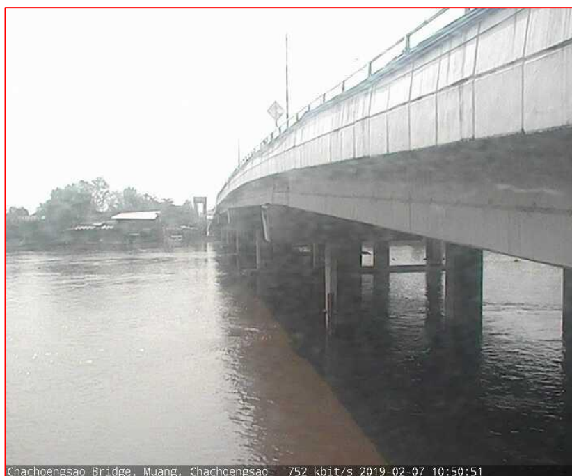
Chachoengsao Bridge, Muang, Chachoengsao 752 kbit/s 2019-02-07 10:50:51
