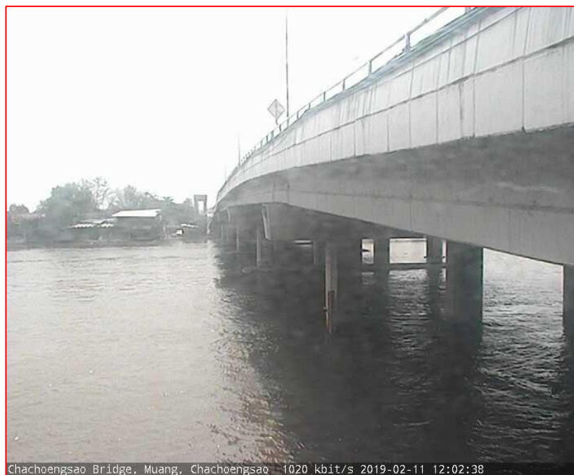
Chachoengsao Bridge, Muang, Chachoengsao 1020 kbit/s 2019-02-11 12:02:38
