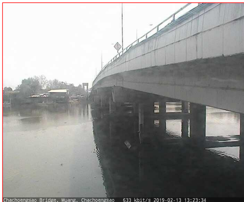
Chachoengsao Bridge, Muang, Chachoengsao 633 kbit/s 2019-02-13 13:23:34
