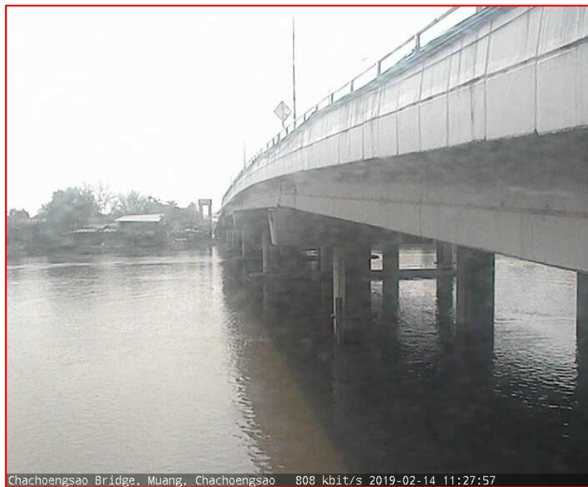
Chachoengsao Bridge, Muang, Chachoengsao 808 kbit/s 2019-02-14 11:27:57
