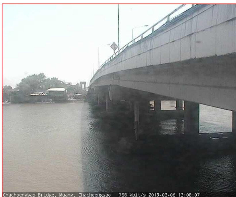
Chachoengsao Bridge, Muang, Chachoengsao 768 kbit/s 2019-03-06 13:08:07
