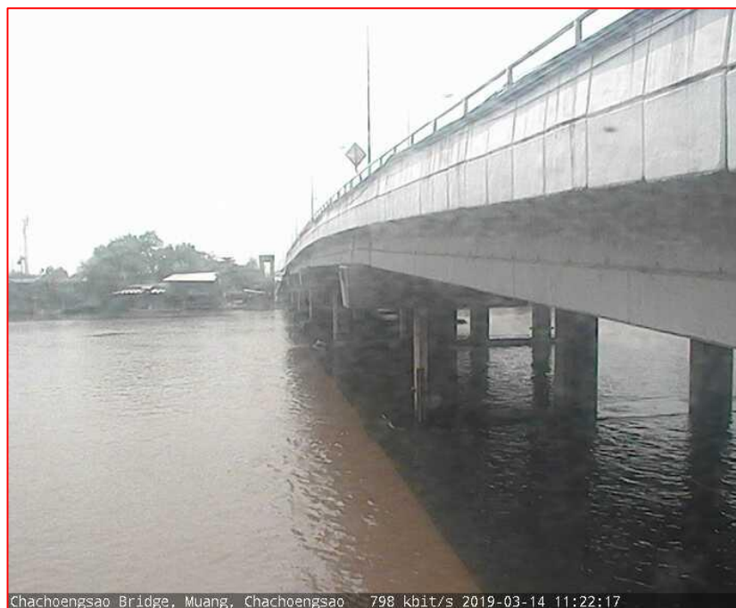
Chachoengsao Bridge, Muang, Chachoengsao 798 kbit/s 2019-03-14 11:22:17
