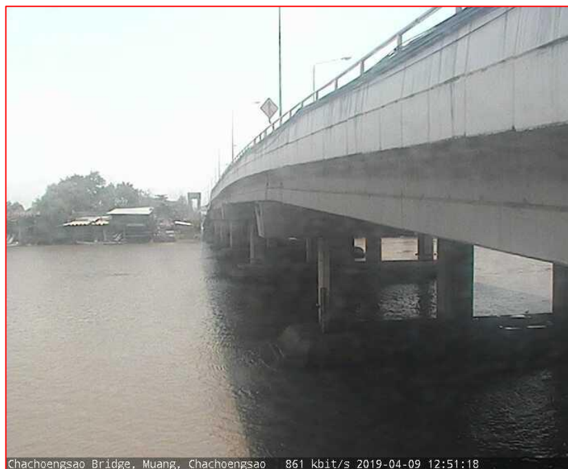
Chachoengsao Bridge, Muang, Chachoengsao 861 kbit/s 2019-04-09 12:51:18
