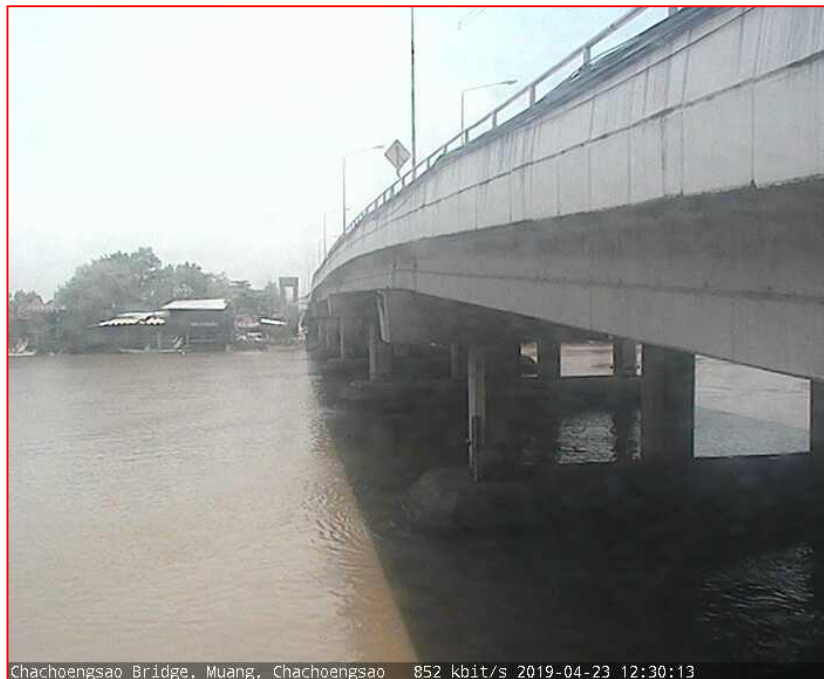
Chachoengsao Bridge, Muang, Chachoengsao 852 kbit/s 2019-04-23 12:30:13
