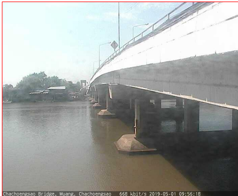
Chachoengsao Bridge, Muang, Chachoengsao 668 kbit/s 2019-05-01 09:56:18
