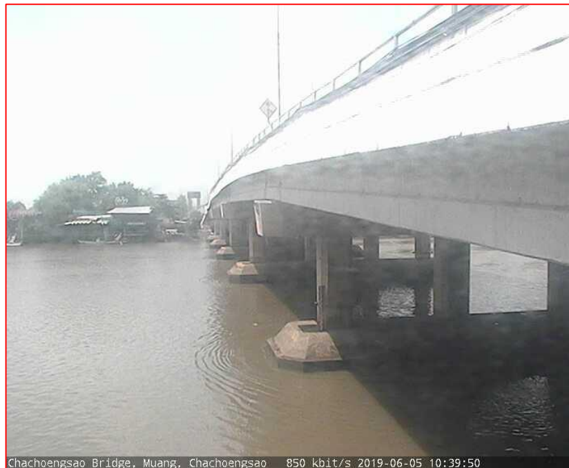
Chachoengsao Bridge, Muang, Chachoengsao 850 kbit/s 2019-06-05 10:39:50
