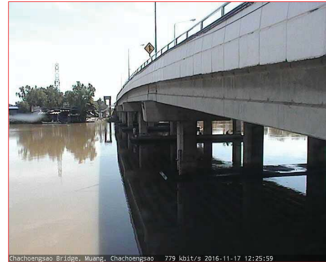
Chachoengsao Bridge, Muang, Chachoengsao 779 kbit/s 2016-11-17 12:25:59
