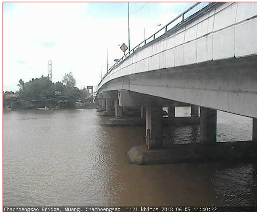
Chachoengsao Bridge, Muang, Chachoengsao 1121 kbit/s 2018-06-05 11:40:22
